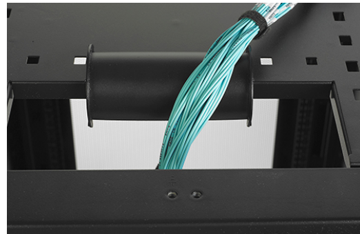
Installed on rear roof hole of AR3100
